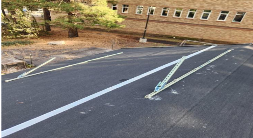
Figure 33: Panel Mounting Assembly
