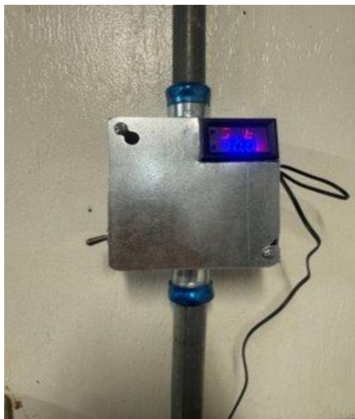
Figure 36: J-box with Thermostat and Switch
