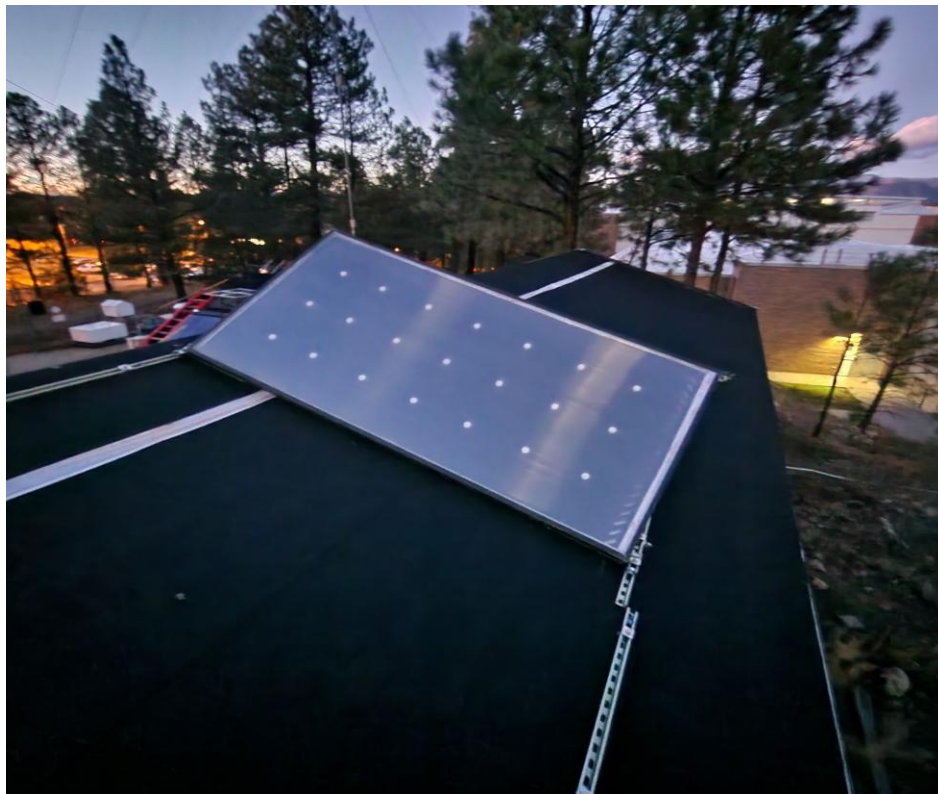
Figure 34: Mounted Angled Solar Panel
