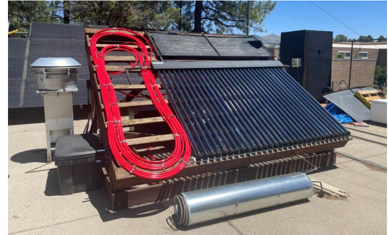
Figure 7: Closed Loop Solar Water Heater
