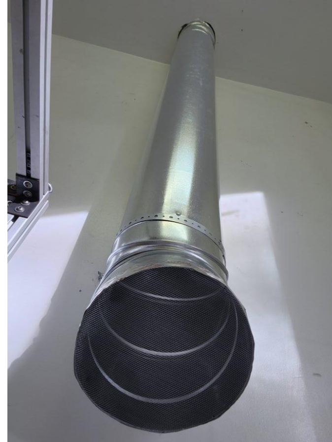
Figure 33: Input Duct for Front Room
