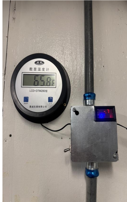
Figure 35: Master Switch and Thermostat
