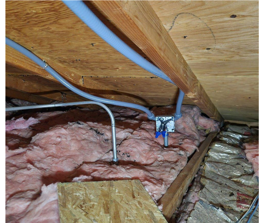
Figure 36: Conduit Through Attic
