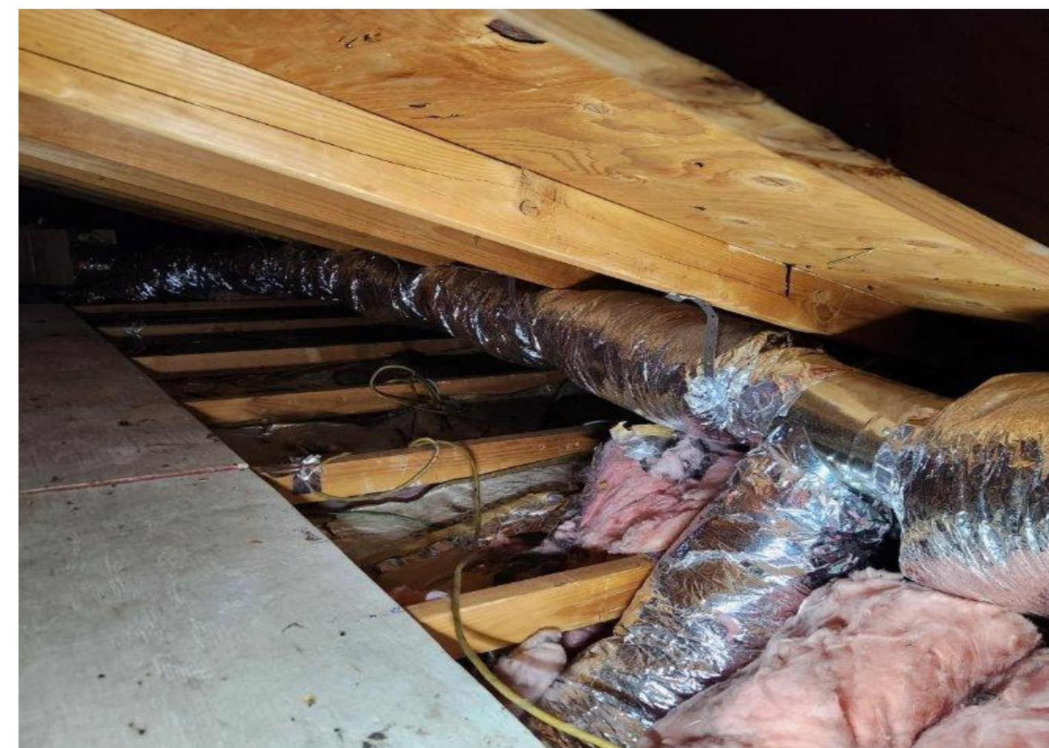
Figure 1: Duct Work Throughout Ceiling
