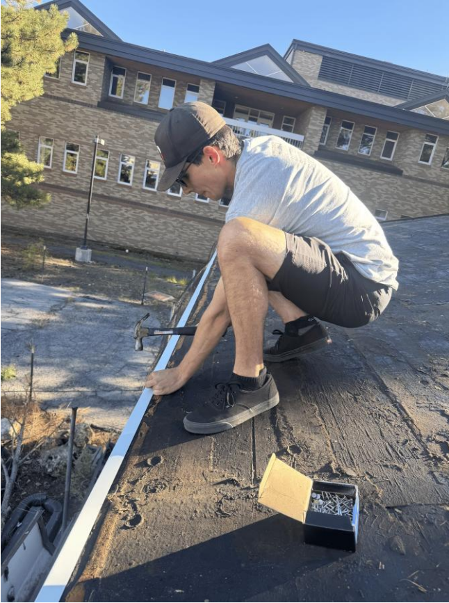
Figure 12: Applying Drip Edge Flashing
