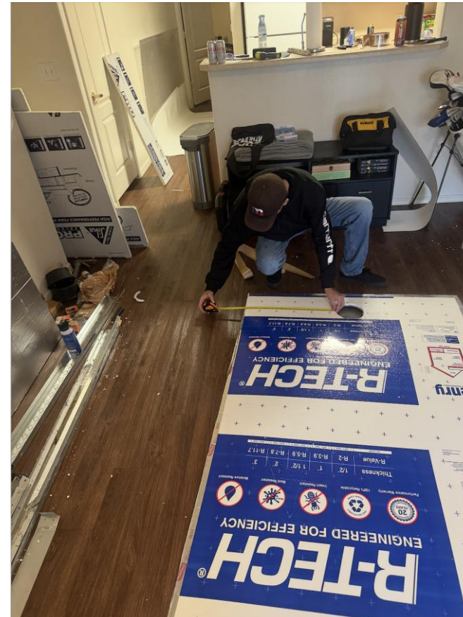
Figure 16: Replacing Insulation
