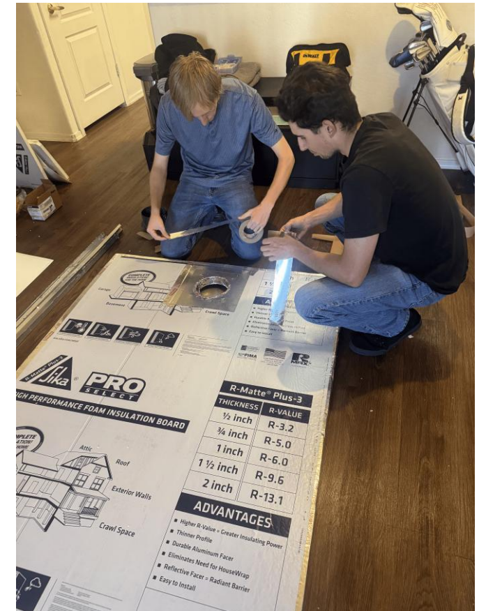
Figure 17: Applying Tape to Edges
