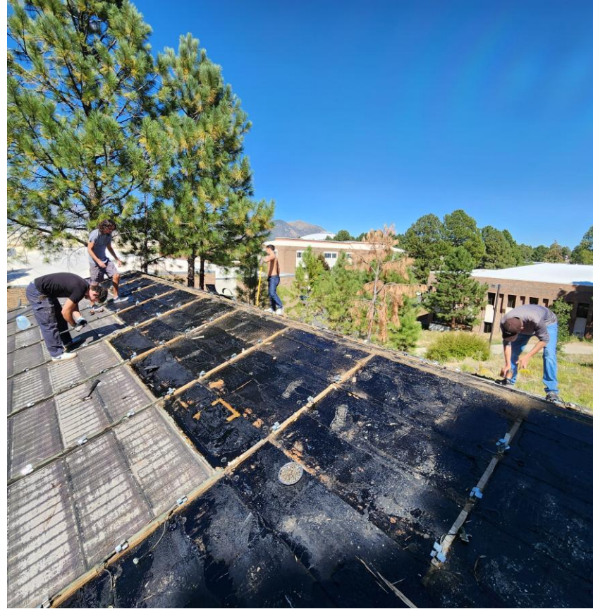
Figure 9: PVT Panel Removal
