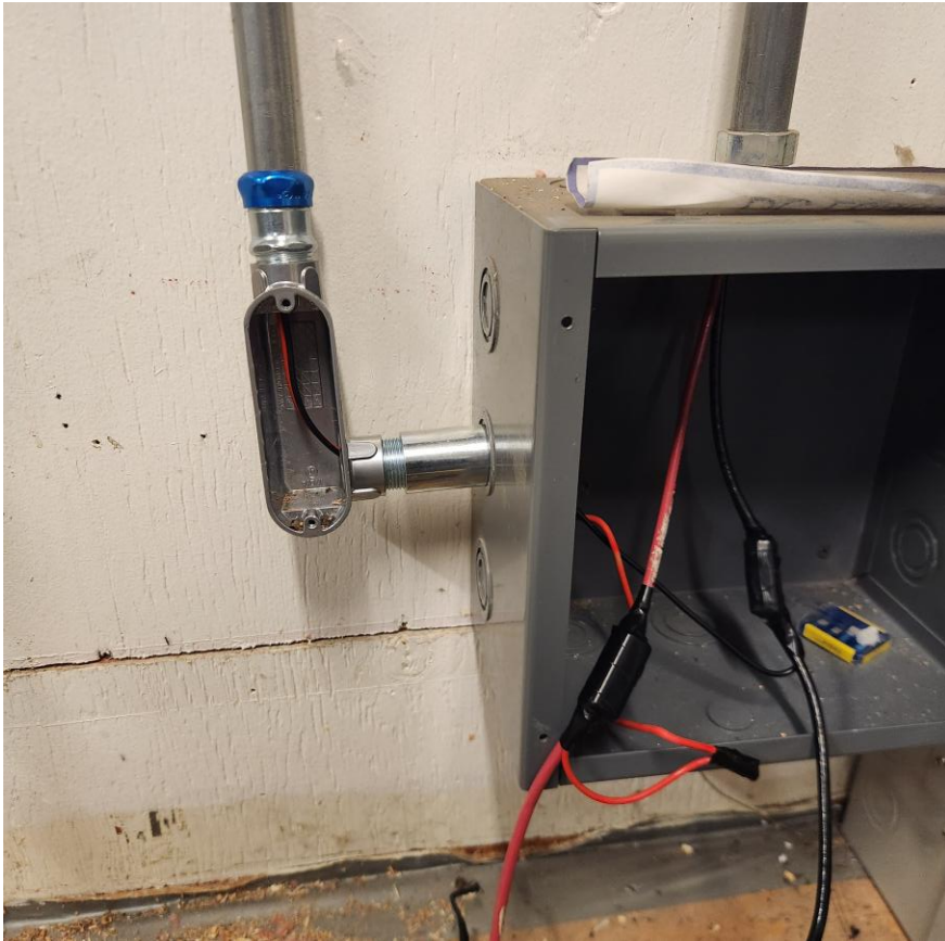
Figure 13: Load Box Wiring
