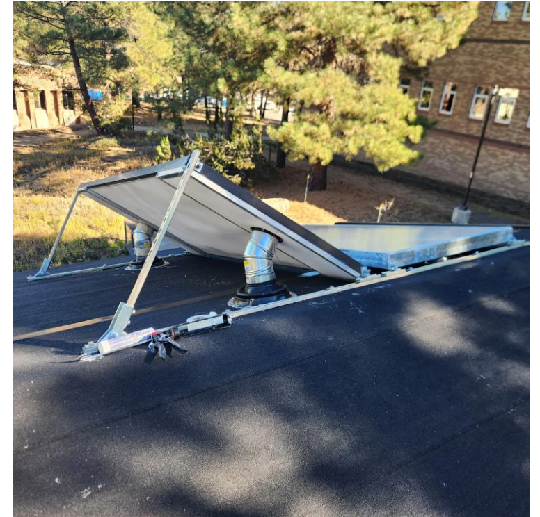
Figure 9: Mounting Installation
