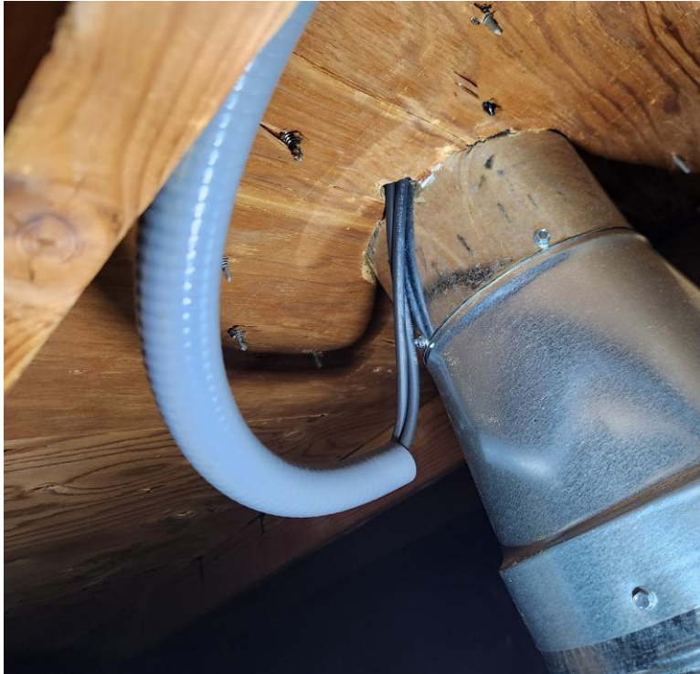
Figure 15: Conduit to Flat Solar Panel
