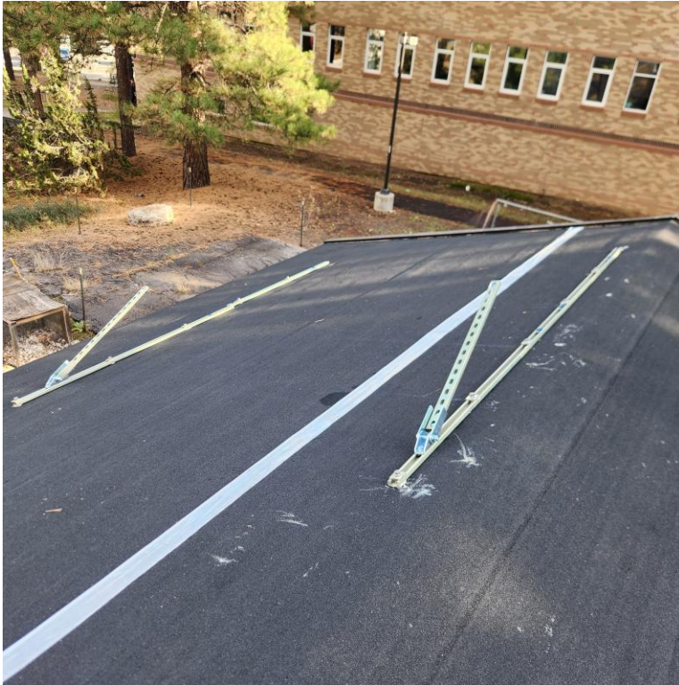
Figure 7: Mounting Unistrut
