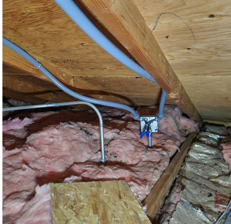
Figure 16: Splitting Wires for Fans
