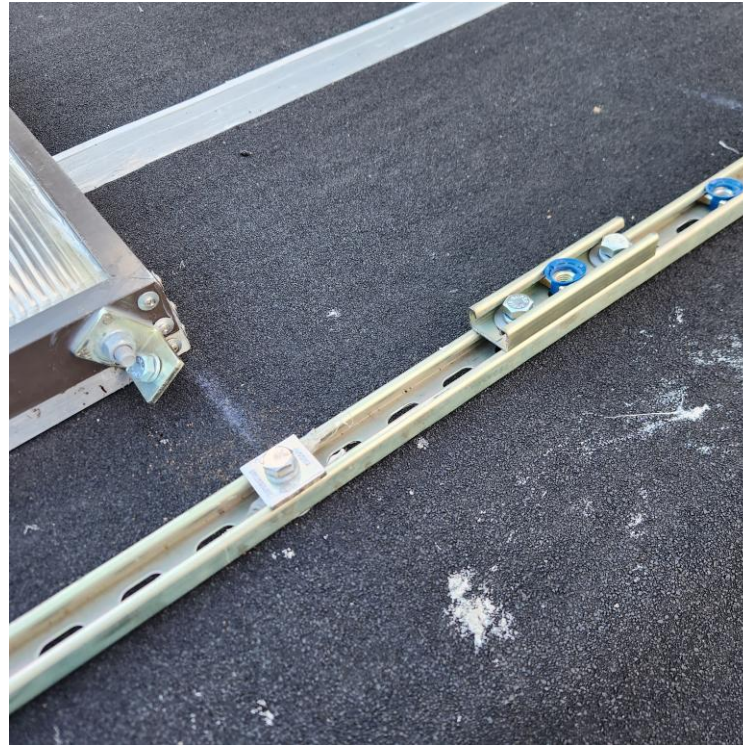
Figure 8: Making Adjustment to Unistrut
