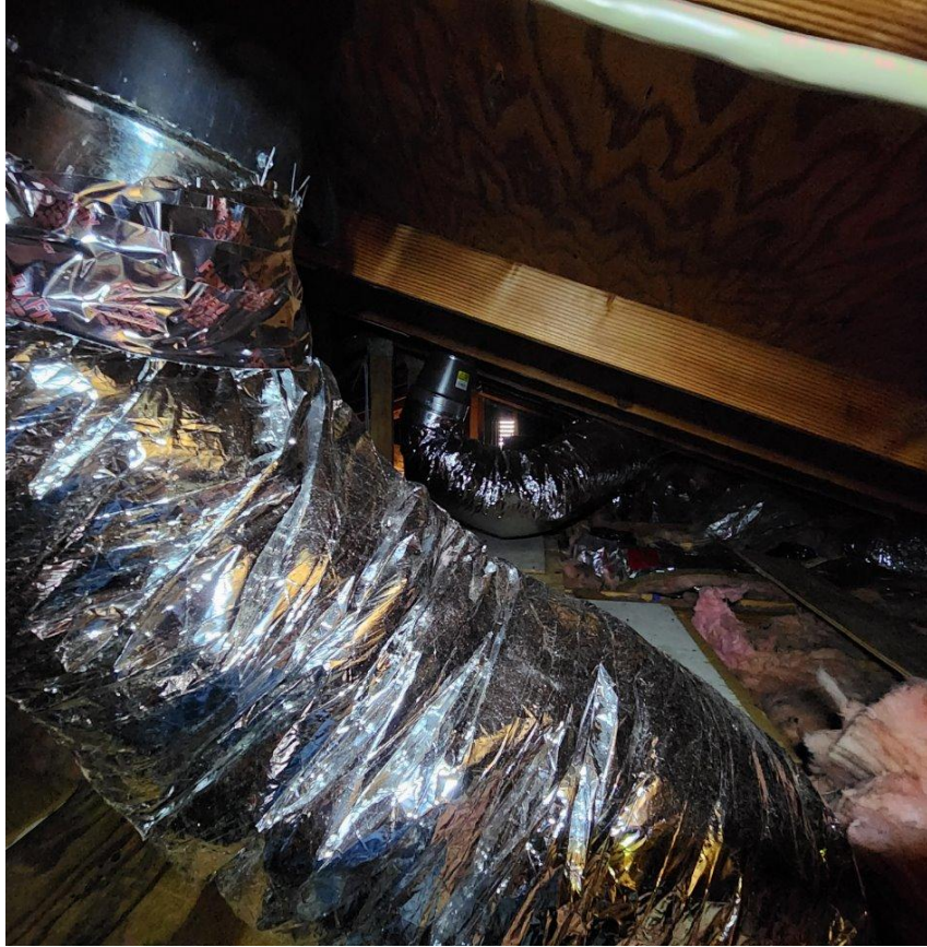
Figure 18: Hot Air into Attic
