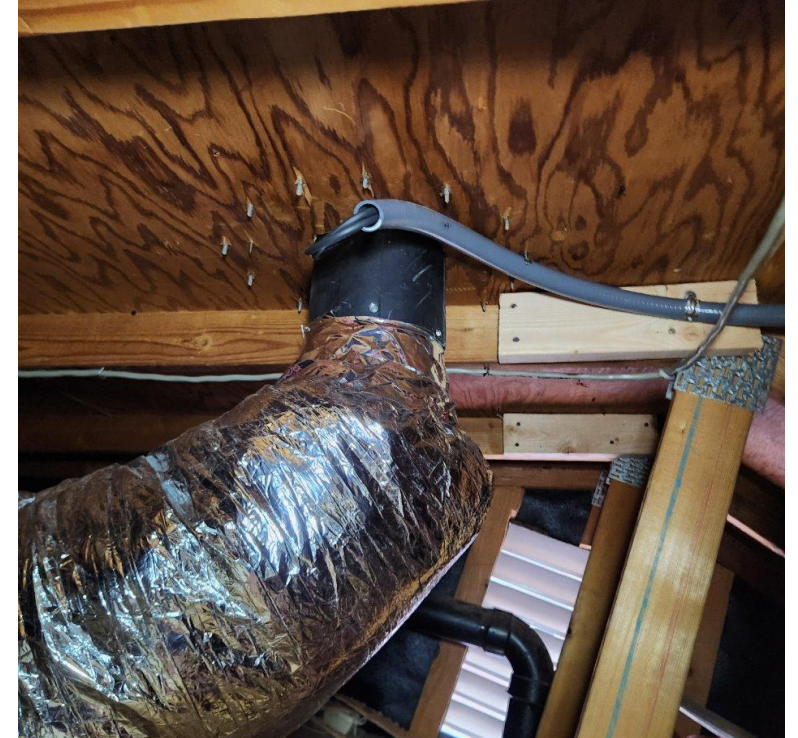
Figure 17: Conduit to Inclined Solar Panel
