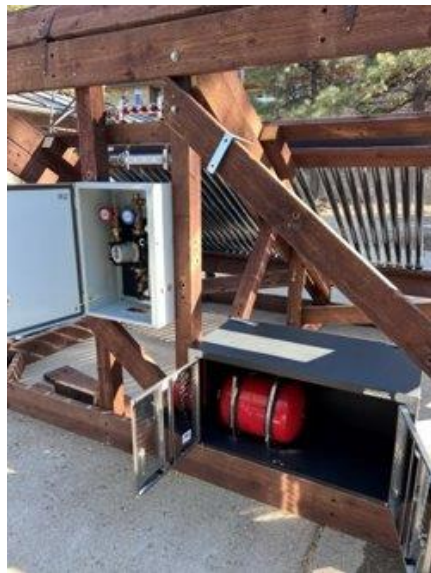
Figure 10. Expansion tank and general storage.
