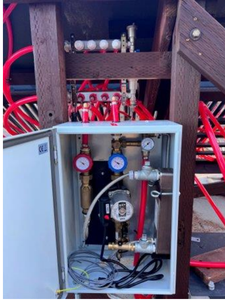
Figure 9. Pumpstation, manifold, and heat exchanger
