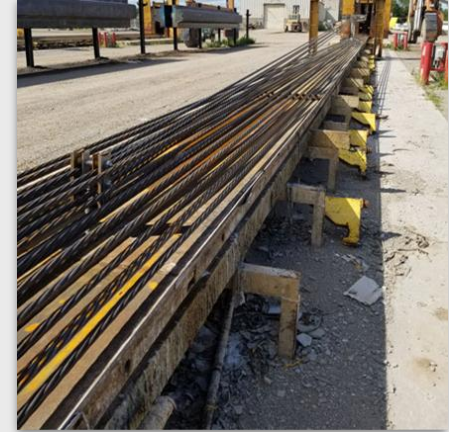
Figure 7: Pre-tension Casting Bed [6]
