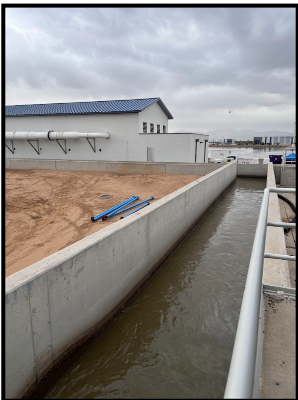
Photo 3: Open channel flow after headworks
