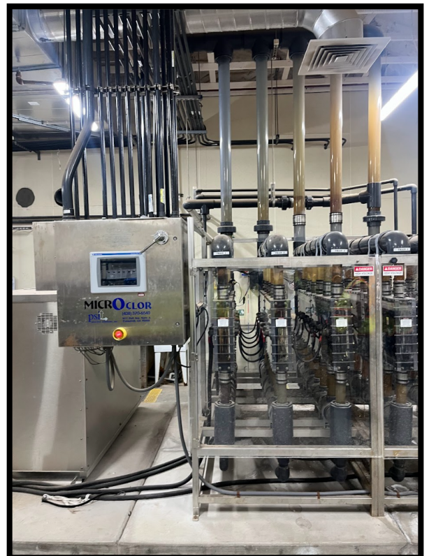
Photo 8: Microchlor onsite hypochlorite generator
