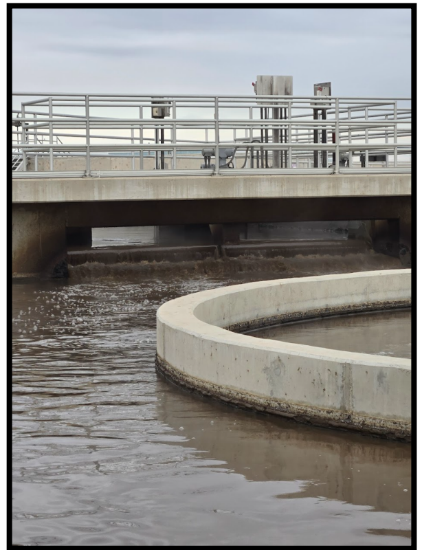
Photo 6: Flow entering Plant 5 over a weir
