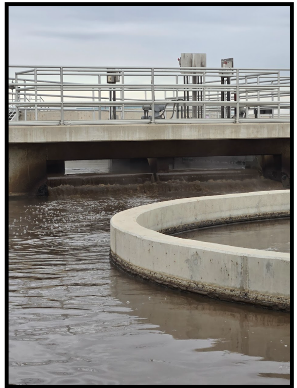
Photo 6: Flow entering Plant 5 over a weir
