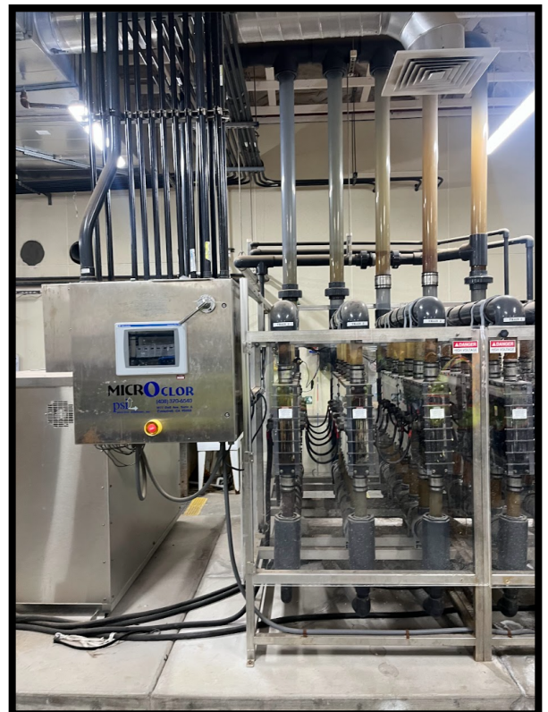
Photo 8: Microchlor onsite hypochlorite generator
