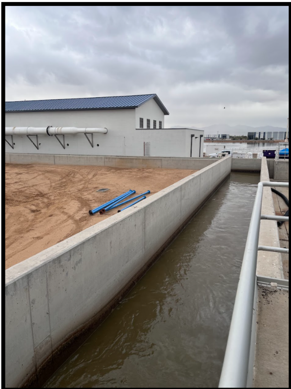
Photo 3: Open channel flow after headworks
