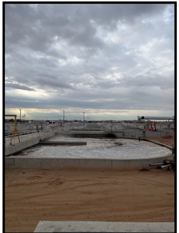
Photo 4: Plant 3 Oxidation Ditch
