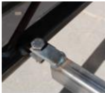
Figure 3-13: Connection 3 - Straight Cross Bracing
