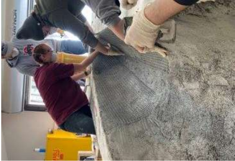
Figure 18: Reinforcement Placement
