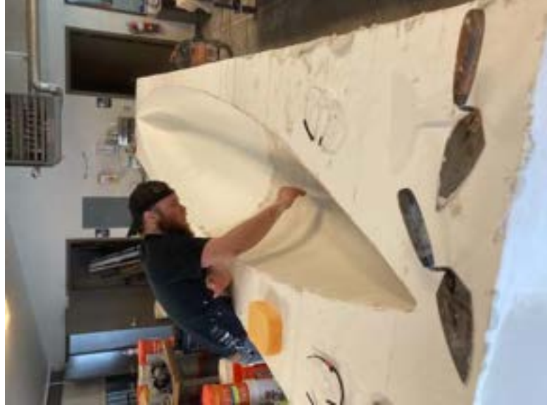
Figure 16: Drywall Application
